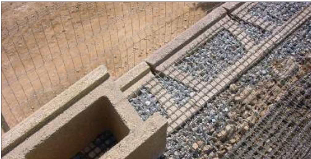
Allan Block reinforced with Huesker geogrid.
