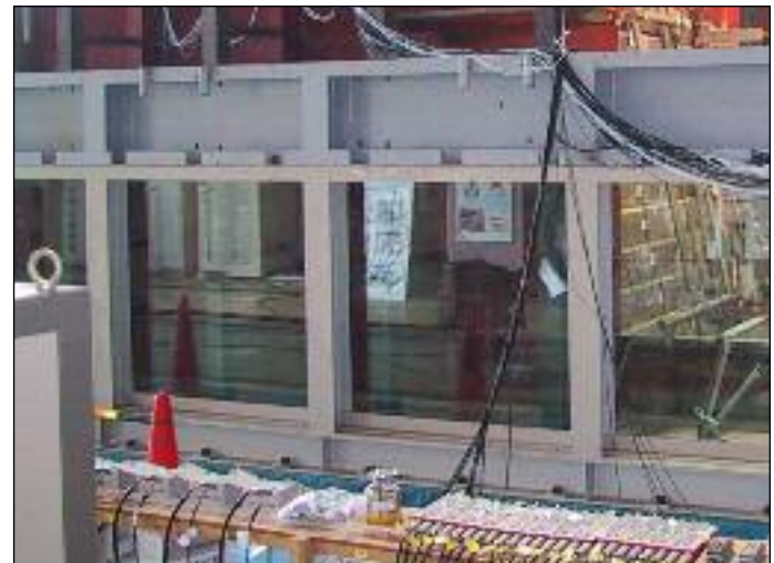
Steel Container for Wall Construction
