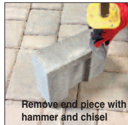
Flip the AB York block over below end cap
